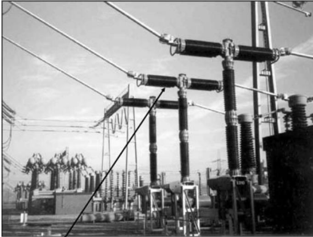
Contacts and arc-quenching mechanism
